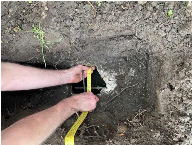
Figure 1 – 29inches / 74 cm from Rebar to internal chamber wall # 1
