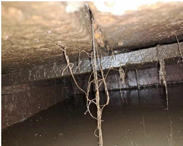
Figure 3 - Chamber wall 1 LHS – wall is resting on this lintel and concrete cover.
