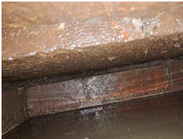
Figure 6 - Chamber wall 1-2 corner
