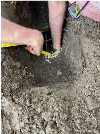
Figure 2 - 15 inches/38cm from rebar to chamber wall 2
