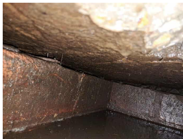
Figure 8 - Chamber wall 3 - 4 corner
